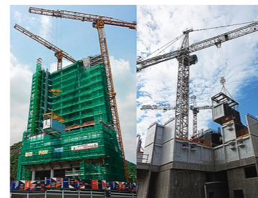
High-rise Modular Integrated Construction (Courtesy of HKSTP and ArchSD)
